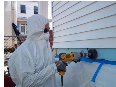
Weatherization Technician prepares home to receive sidewall insulation measures.
