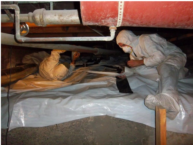
Weatherization technicians work on installing insulation measures into a basement crawlspace.
